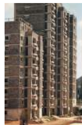
14 storey skyscraper Nuremberg (Germany)
