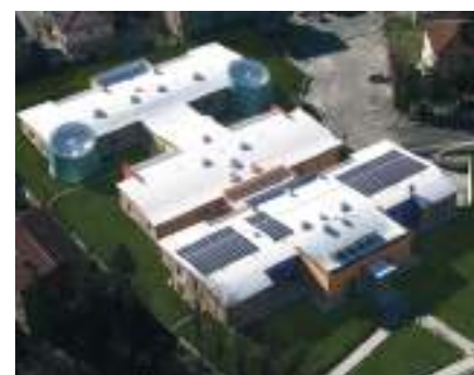
Pavullo school complex (MO) - Italy
