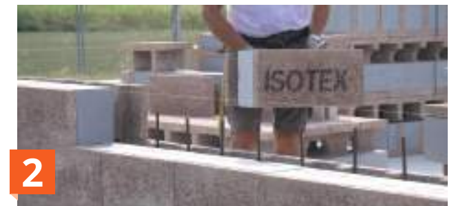
All subsequent rows laid dry
