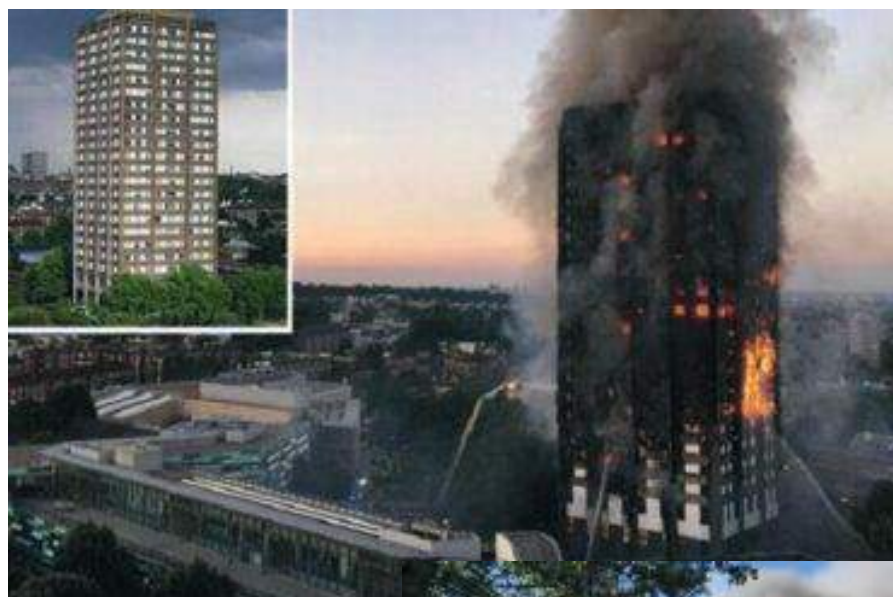
Grenfell Tower London - 2017
