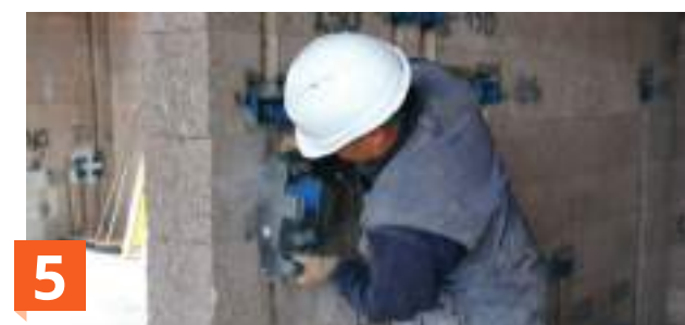
Chasing of wall with a router
