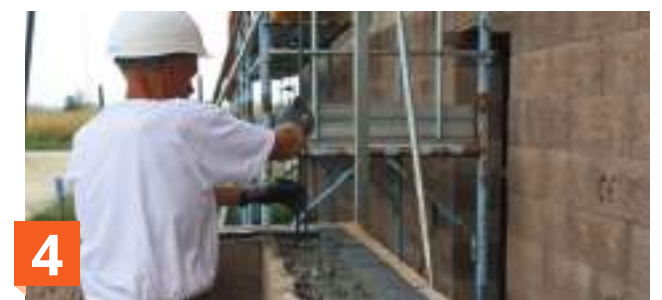
Fresh casting insertion of vertical seismic steel reinforcements
